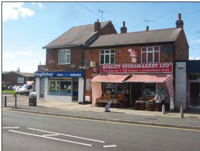
Retail units to the west of the retail area
