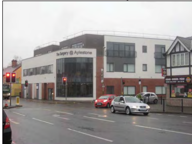
New health centre and retail units, Aylestone Road
