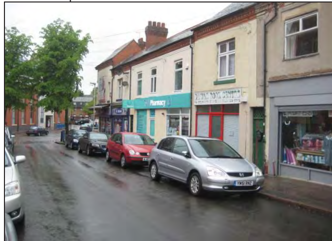
Row of shops at Berners Street
